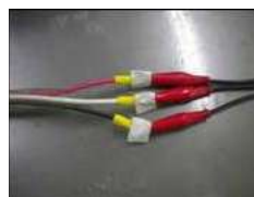
Fig. 2-7 Clip covered with insulation tape
